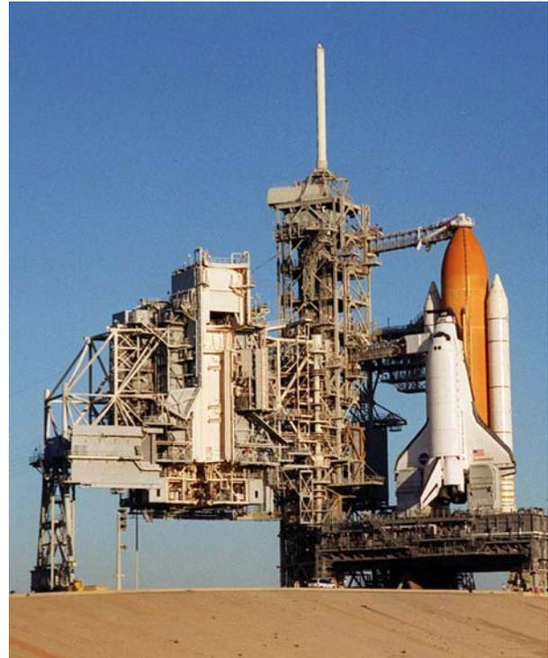
The Rotating Service Structure after rollback to the park position prior to launch of the STS-97 Shuttle Mission. (Image: NASA)
